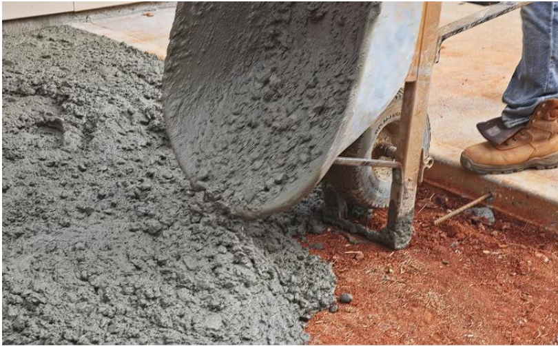
Figure 4. Placement in slabs
